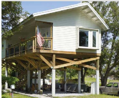
The Patty's House (above) follows the model of a dog-trot, a southern vernacular house type. The design addresses the challenges of an elevated house. The house is thirteen feet off the ground to meet the FEMA advisory flood elevations. The house structure is innovative with a combination of concrete and pressure treated wood.
