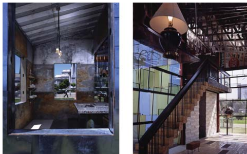
Public Architecture led the design and construction of "Scrap House," a temporary demonstration home, built entirely of salvaged material (above). Walls were sheathed with everything from street signs and shower doors.
